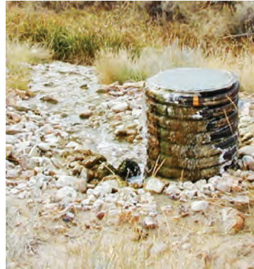
Oil and gas discharge outfall of produced water.
