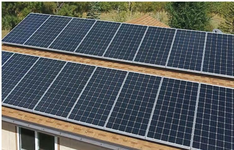
they have installed. Modern panels are predicted to last anywhere from 30-50 years, payback time is less than 10 years for most systems, and savings are both environmental and financial.
