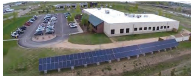
A 27 kW Pole Mounted Photovoltaic system in Wyoming that received a REAP Grant.
