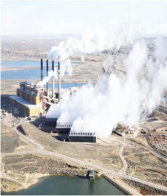
The Jim Bridger Power Plant near Rock Springs
