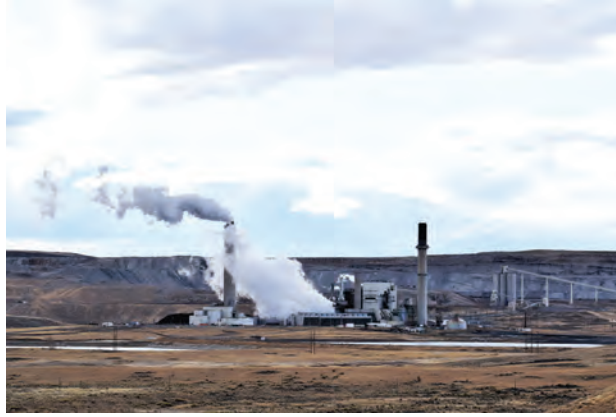
Ash ponds at the Naughton power plant in Kemmerer.
