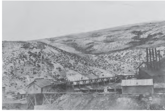
The Kemmerer Coal Mine in the early 1900s. Photo from the Diamondville Miners' Memorial Park.
