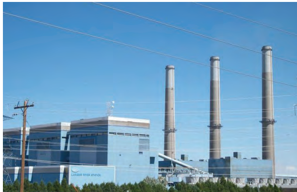
Laramie River Station Coal Plant
