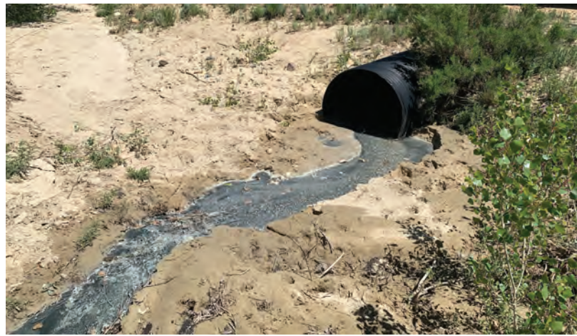
A source of Aethon wastewater discharge. (Photo from Wyoming DEQ)
