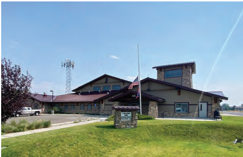
Laramie’s Fire Station #3
