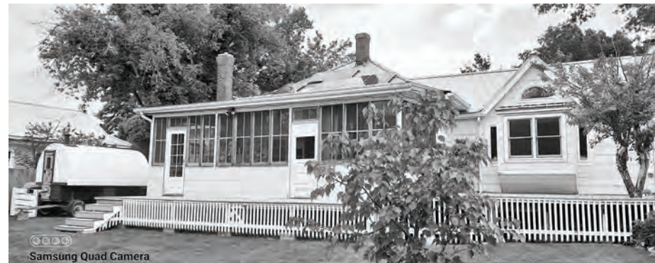
Solar panels on David and Margo's home
