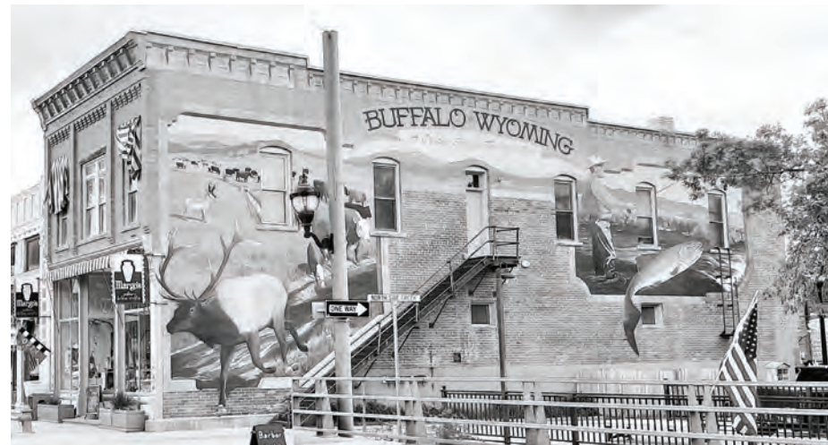
The solar panels on Margo's Pottery aren't visible from the ground but they are helping power this historic building on Buffalo's Main Street.
